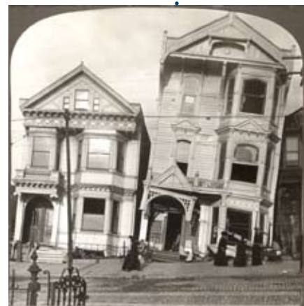
"After the earthquake—frame houses tumbled from their foundations, San Francisco Disaster, U.S.A." (1906) Library of Congress
