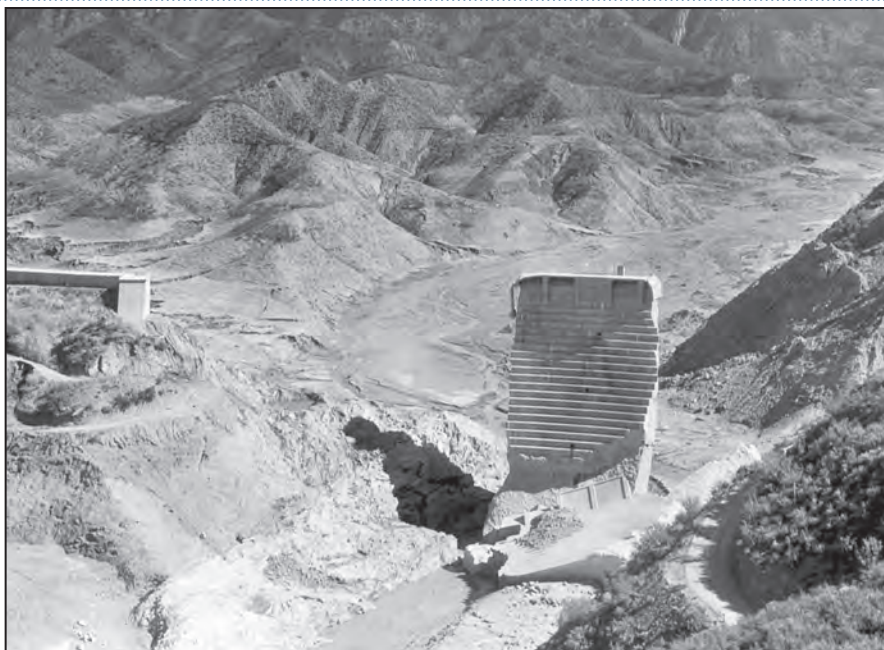
The collapse of the St. Francis Dam on March 12, 1928, swept away ranches, homes and businesses, leaving more than 450 people dead. It ranks as California's second most deadly disaster. USGS
